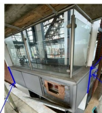
Vertical closed state cavity barrier at the edge of the building to separate the balcony.
